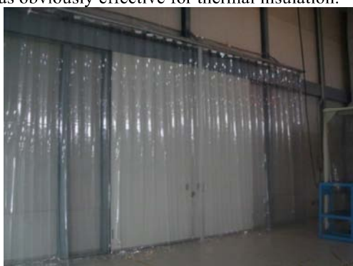
Fig. 3. A thermal insulated curtain at a carrying door in the experimental hall.
