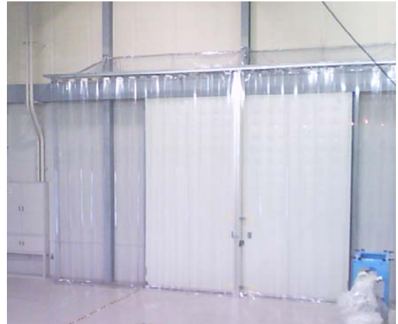
Fig.2 Shield curtain set at the service entrance.
